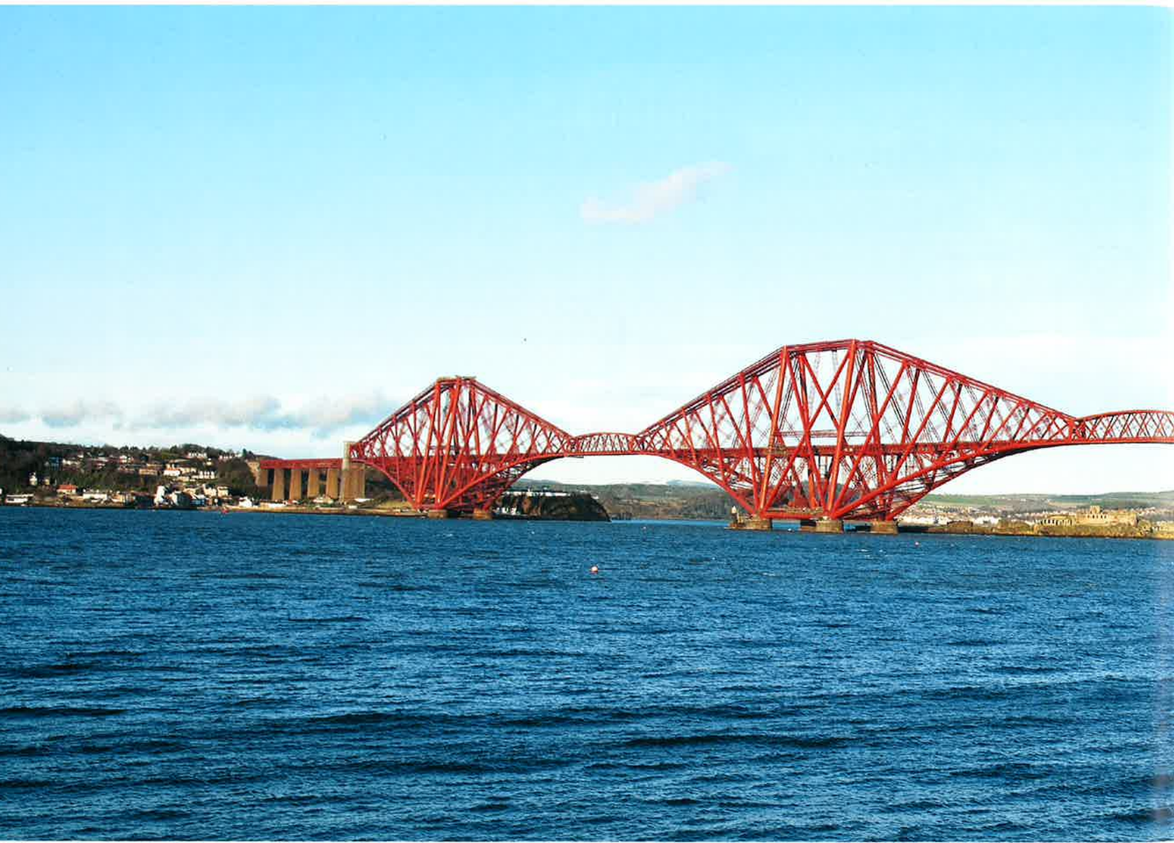
The impressive Forth Rail Bridge was designed by Sir John Fowler and Sir Benjamin Baker in 1879 and serves as a major connection between the Scottish Lowlands and Highlands.
